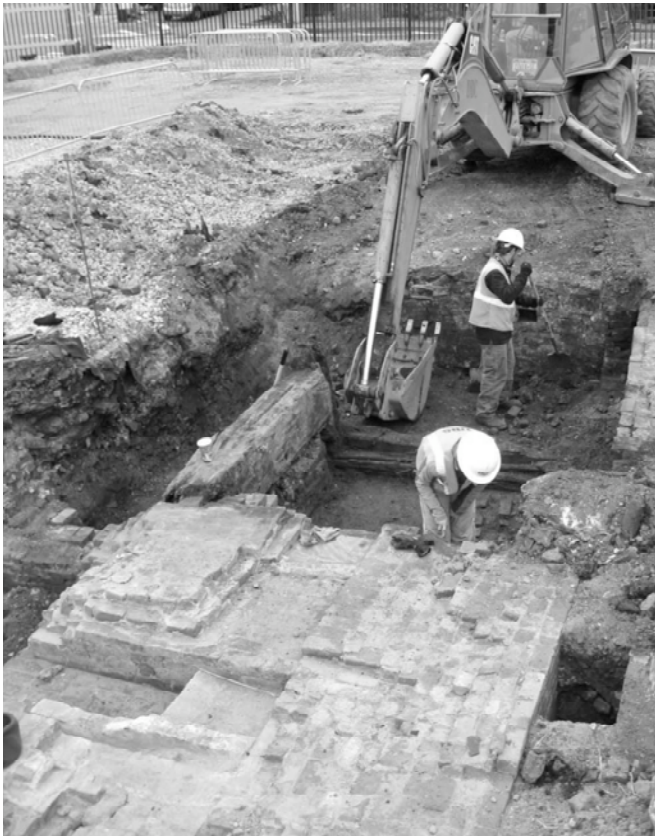
Excavating the foundation remains of the Jewel Flour Mill at the corner of Old Fulton St. and Furman St. Alyssa Loorya and Dan Eichinger, URS Corporation pictured.
