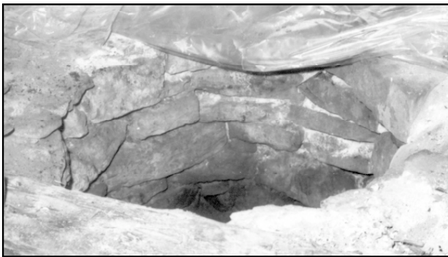
Figure 1: 1966 Photograph of Jessup's well taken during restoration of the 1838 blockhouse. Photo by E. Wylie (2H30X).
