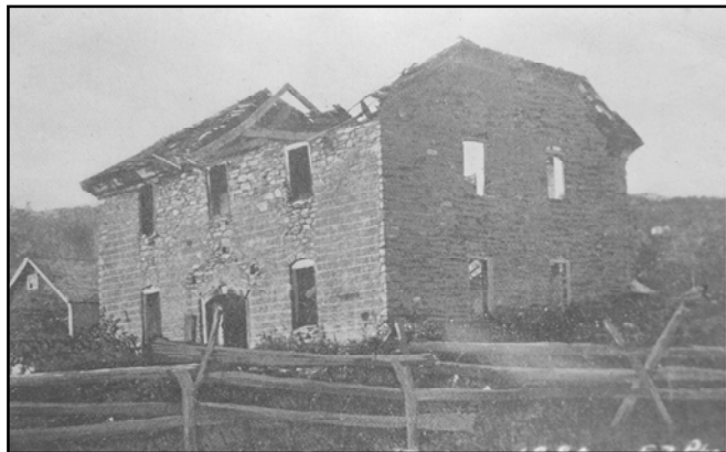
The Old Union Church ruins in Long Valley, Washington Township, New Jersey. Notice the clipped gables on the collapsing roof and the fine stonework façade of the building.
