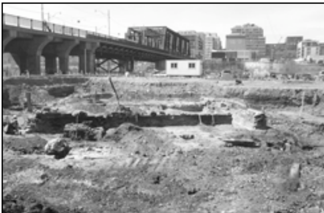
Figure 4. Excavation and documentation of a portion of the 1850s Grand Trunk Engine House in progress.
