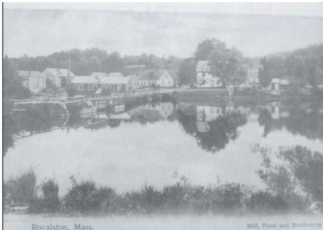
Photo 1. Ca. 1907 postcard showing Newton-Davis Mill complex from across mill pond.
