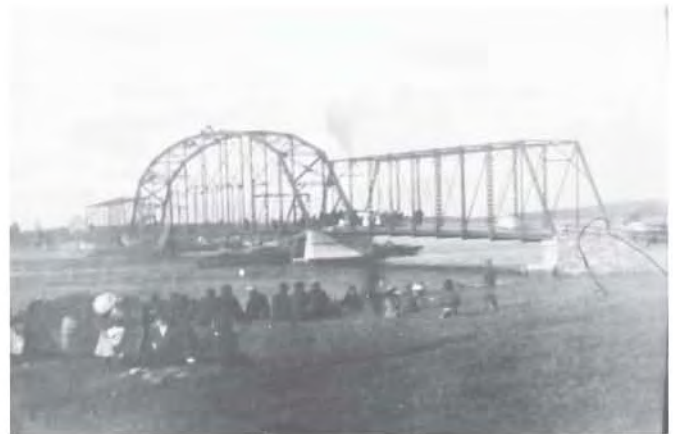
The central section of the Indian Sluice Bridge being floated into place, 1909.
