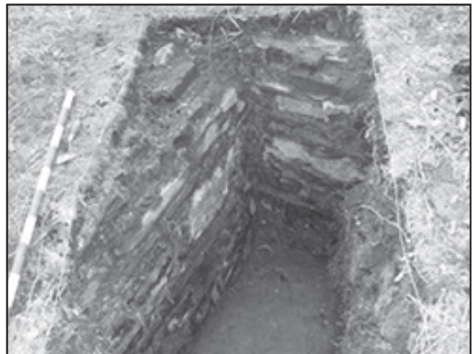
Photo 1. Foundation walls showing brick above stone with wine bottle base in corner.
