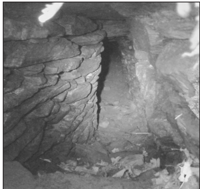
Inside the south tunnel, looking south. Courtesy of production company Left/Right, Inc.
