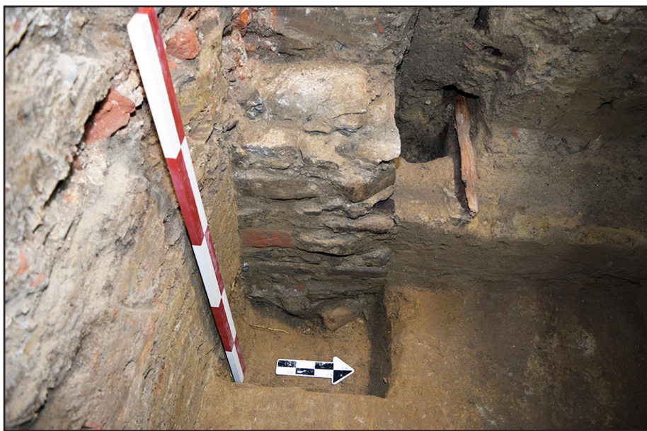
Figure 3: Stone and brick foundation pier associated with the interior courtyard upright structural support posts of the 1831 Market building
