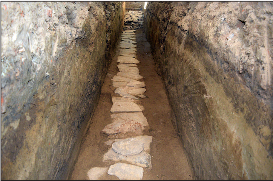
Figure 5: Capstones of the 1831 feeder drain running the length of the trench and meeting the central arched stone drainage sewer visible in the background
