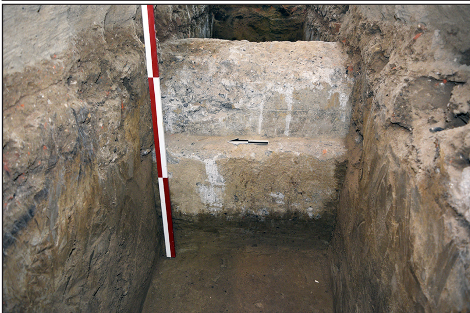
Figure 7: 1904 poured concrete foundation
