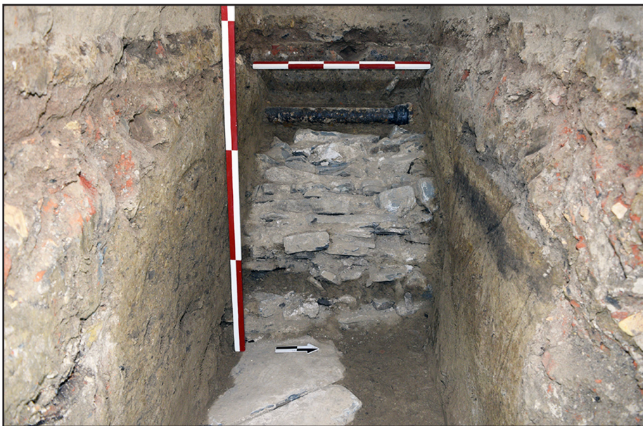
Figure 4: Central arched stone drainage sewer associated with the 1831 Market building, below a modern 4" cast iron utility pipe. The capstones of one of the feeder drains are visible in the foreground
