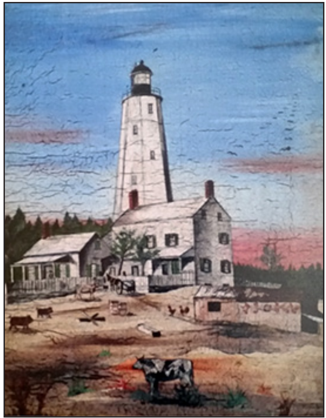
Figure 2. A c. 1870s painting of the Sandy Hook Lighthouse and keeper's dwellings by Frank Paterson. Foundations of both houses were identified in the 2016 excavations.
