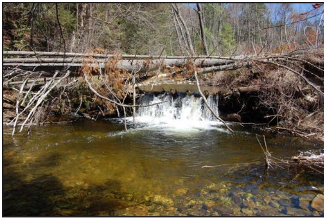
Figure 1. General view of Timber Dam prior to excavation, looking northeast (upstream).
